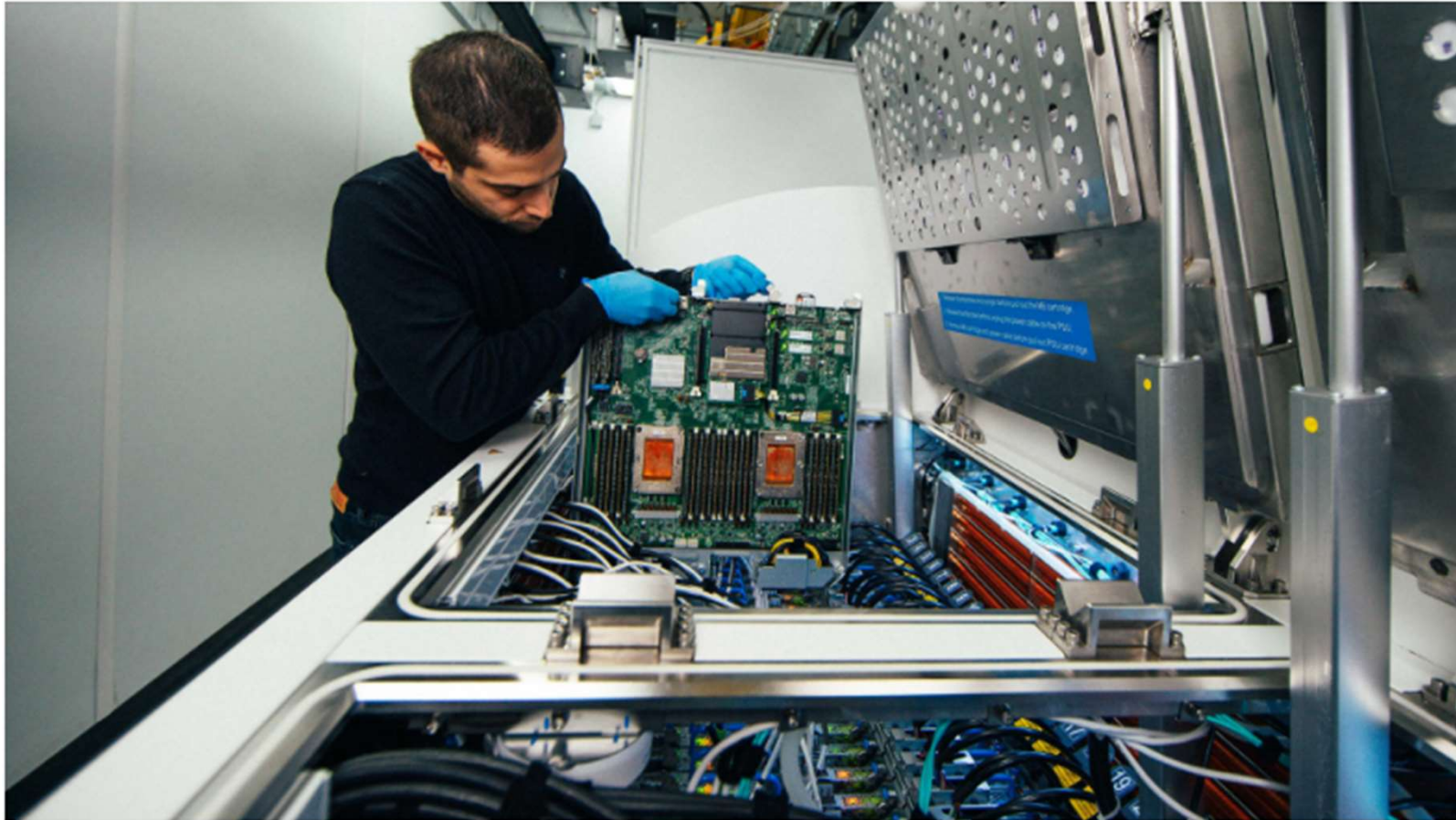
Ioannis Manousakis, a principal software engineer with Azure, removes a server blade from a two-phase immersion cooling tank at a Microsoft datacenter. Photo by Gene Twedt for Microsoft.
